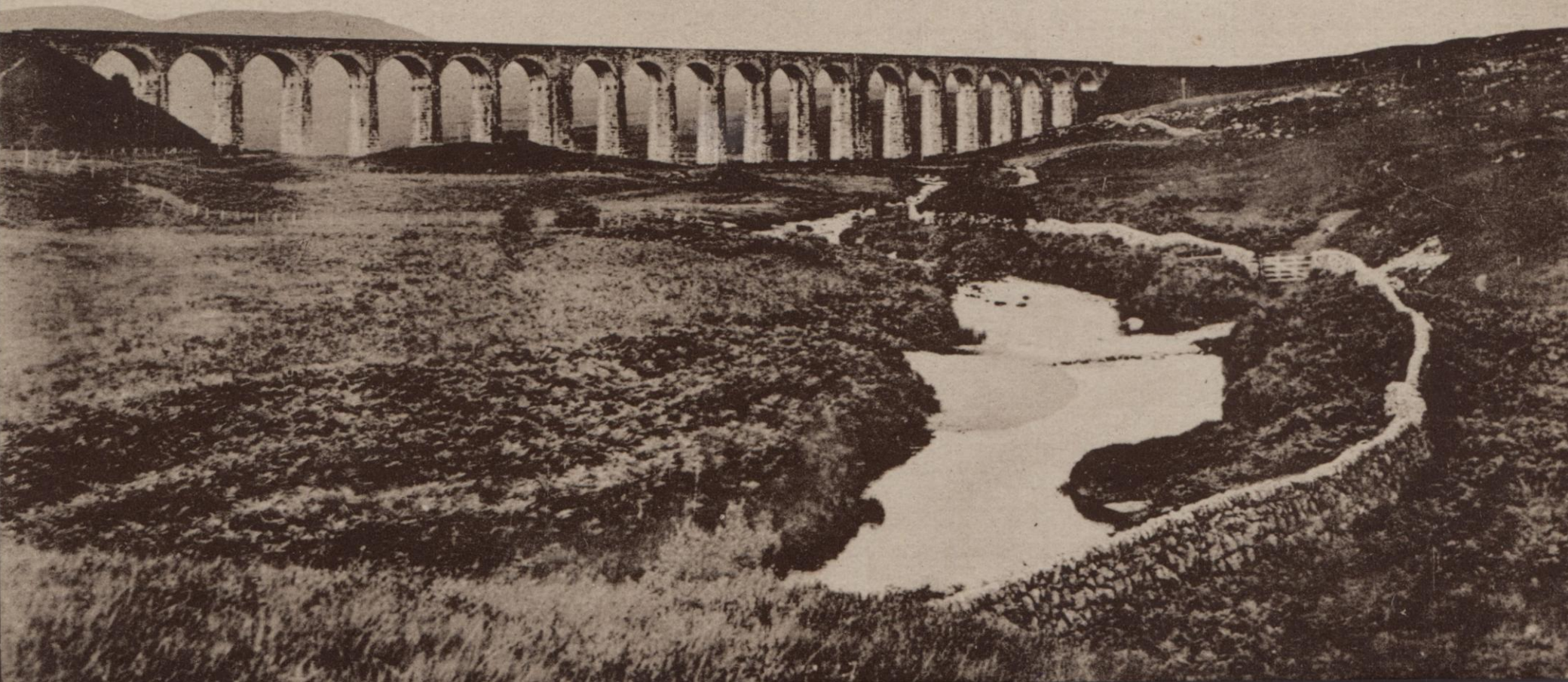
47.010 Big Water of Fleet Viaduct before re-inforcement
